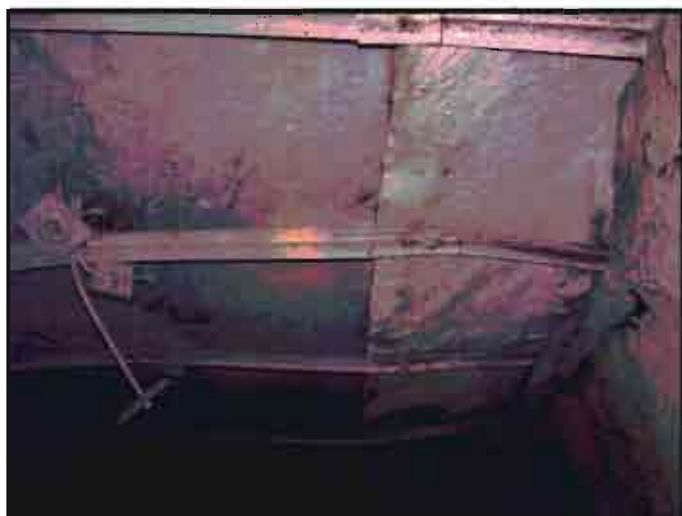
Underground Roof Crack
