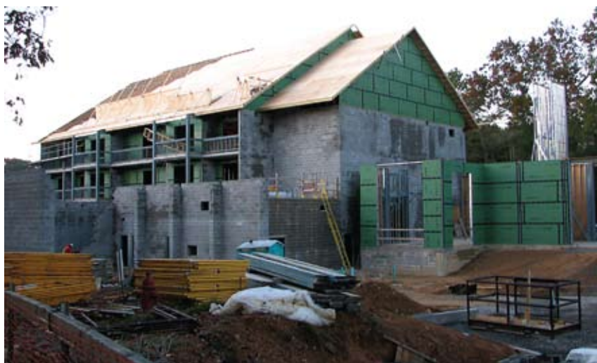
Work on new lodge expansion at Twin Falls Resort State Park.
