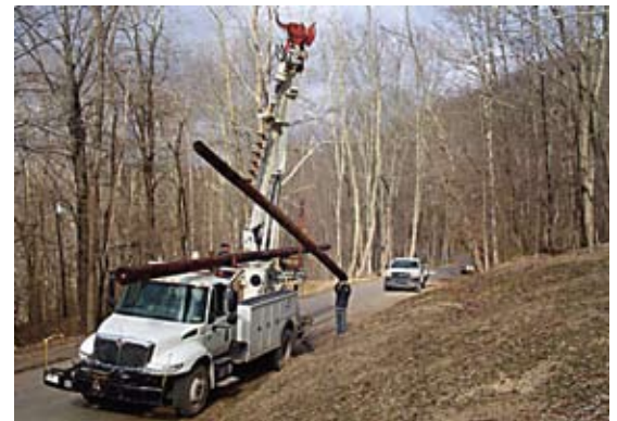
Replacing power lines at Tygart Lake State Park.
