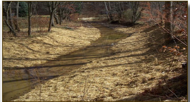
This stream restoration project is located on Little Grave Creek in Marshall County.
