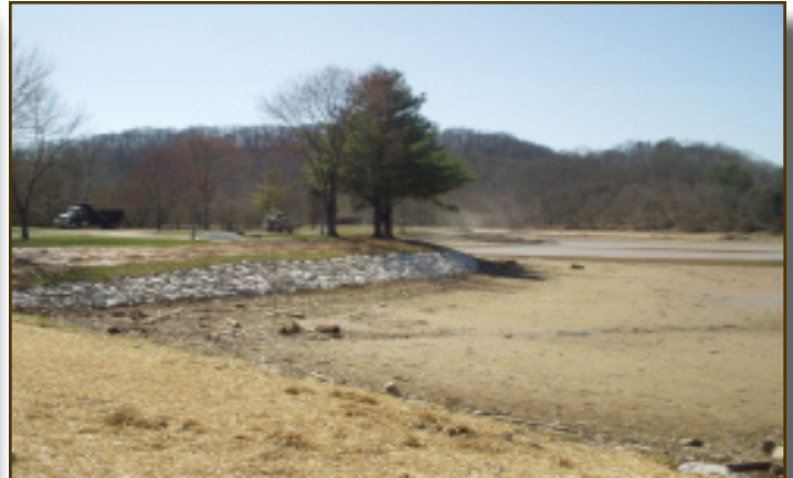
AFTER: 1,000 linear feet of the failing bank was stabilized by incorporating rock rip rap.
