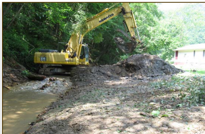
This debris removal crew, contracted by the Guyan Conservation District, works quickly to remove debris from a stream following flooding in Logan County in June, 2010.
