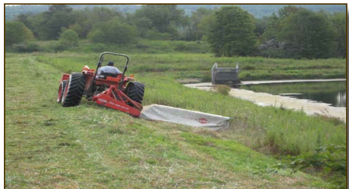
Typical for all dams, this shows brush control maintenance being performed on Upper Deckers Site 6 in Preston County.
