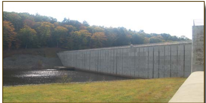
The North fork of the Hughes river is located in Richie County, and is one of only two roller compacted concrete dams in the watershed structure program.
