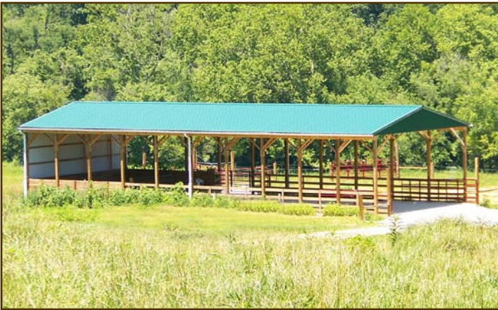
This roofed feeding pad with manure storage structure allows for fewer pollutants to enter streams and groundwater.
