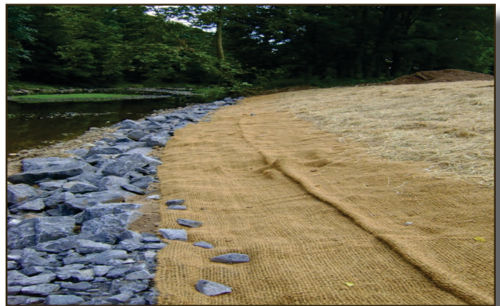
AFTER: WVCA staff used rolled erosion control matting to hold the soil in place and promote vegetative growth.
