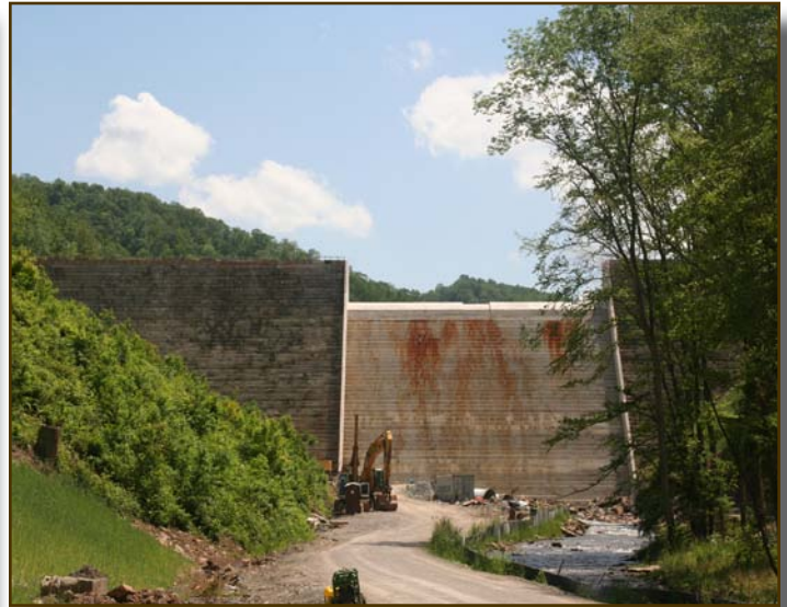
AFTER: The Elkwater Fork Structure, located in Randolph County, is complete and will soon begin holding water.
