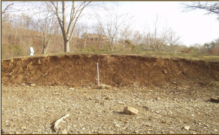
BEFORE: Located in Beech Fork State Park this bank of Beech Fork Lake was severely eroded, increasing sedimentation in the water.
