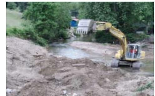
*After the flooding in Logan County, the WVCA and Conservation Districts worked with other agencies to remove debris blockages and to restore floodplains to a more natural state that would allow the streams to hold more water.*
