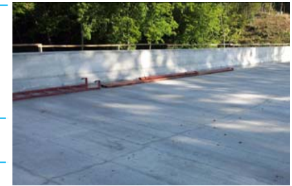
Source: DOH Bridge Inspection Report, Dated 09/30/2014
