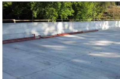
Source: DOH Bridge Inspection Report, Dated 09/30/2014
