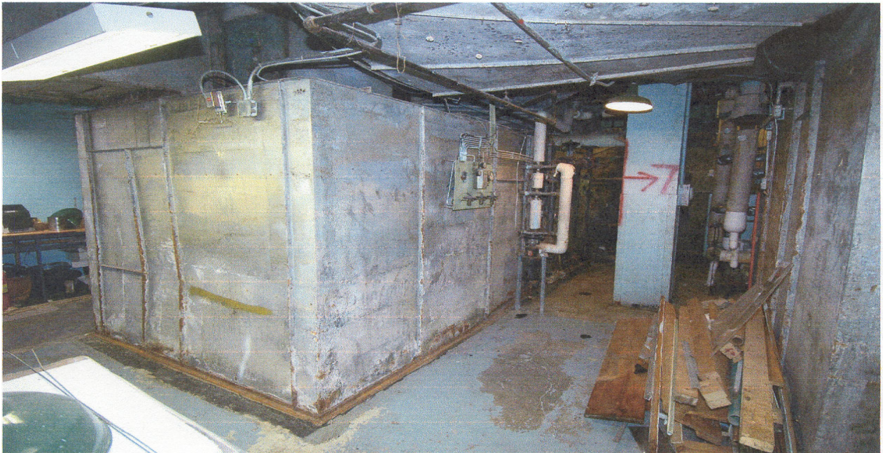
Abestos abatement area for contract #7 in Building 3.
