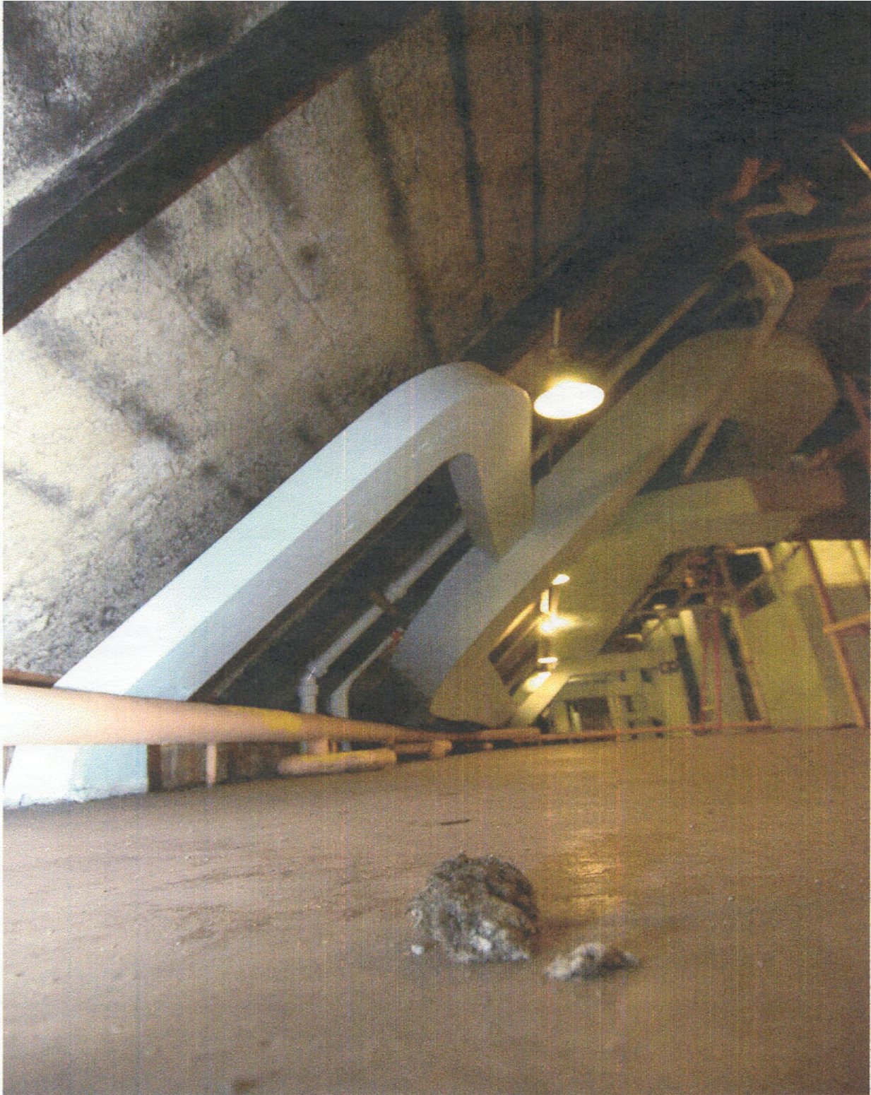
A piece of asbestos fallen from the ceiling in the attic of Building 3.
