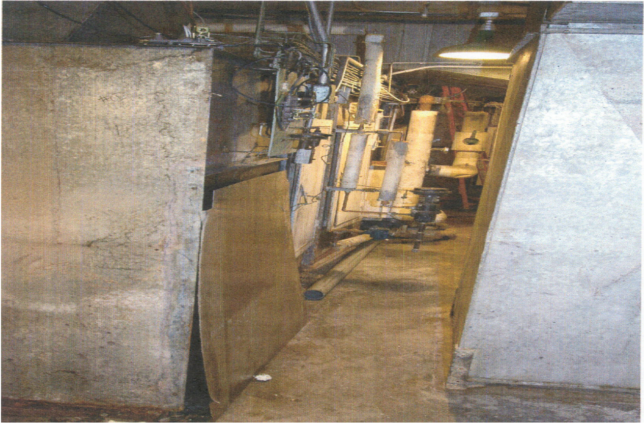
There is a distance of 3 feet between the HVAC Units in Building 3.
