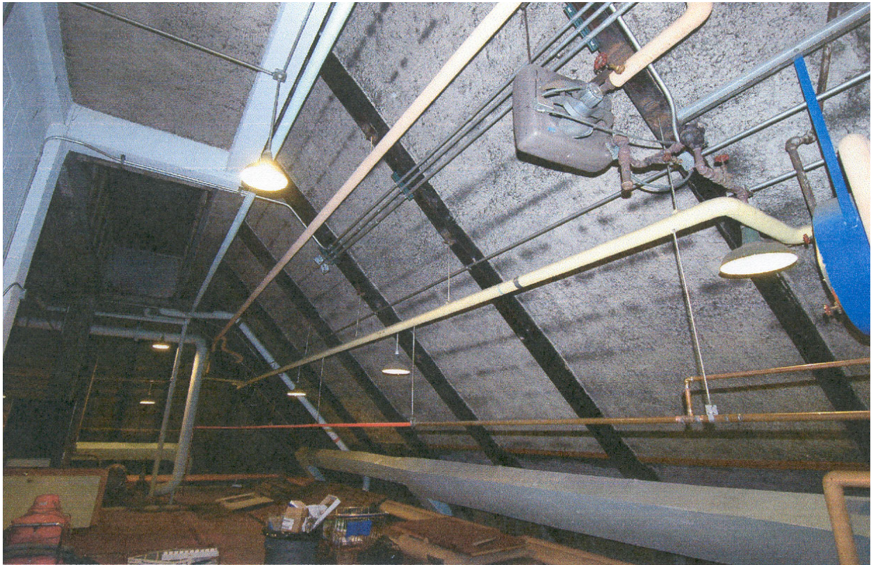
Loose asbestos hanging on walls and ceiling in the attic of Building 3.
