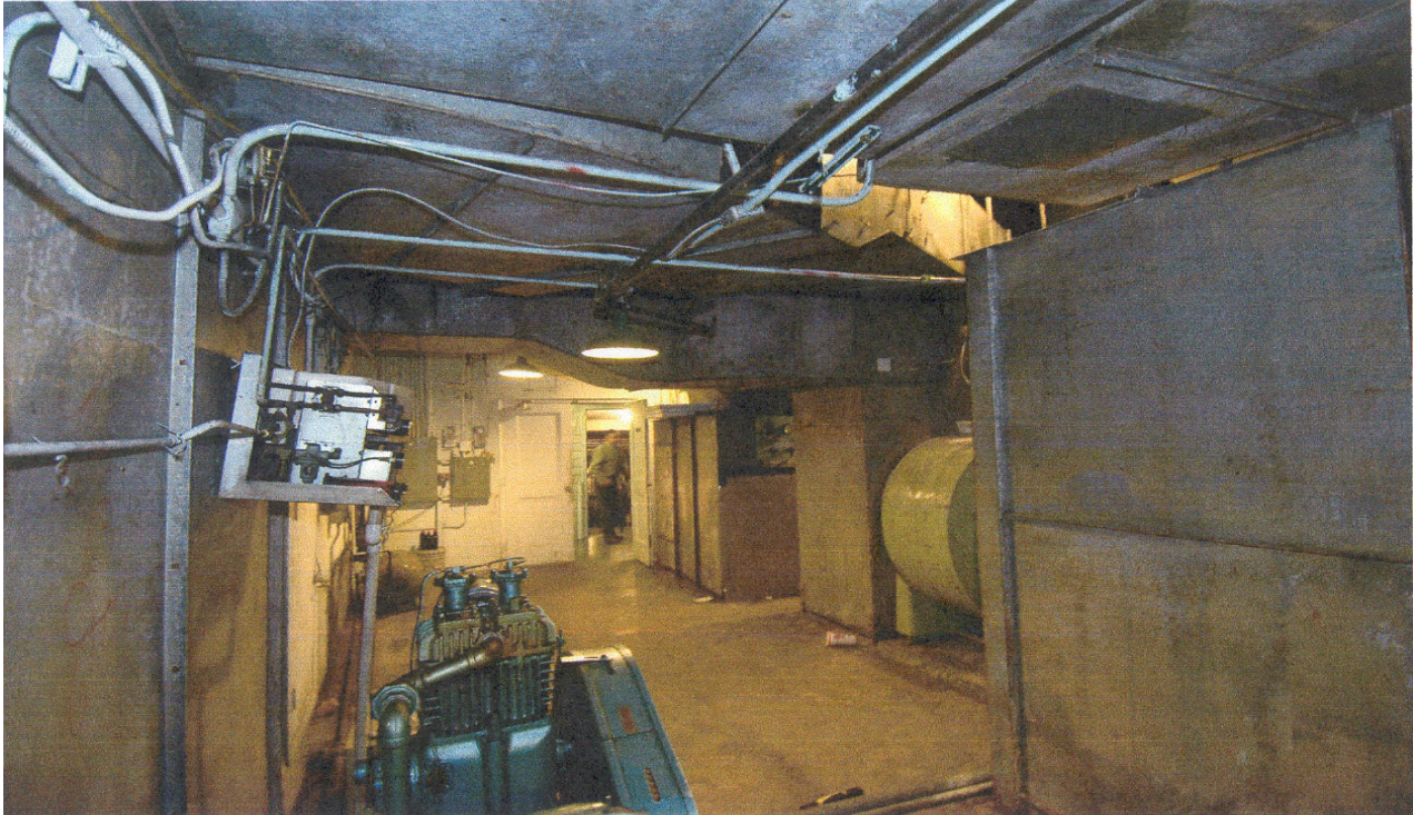
Building 3 HVAC units 1-4 abatement area.
