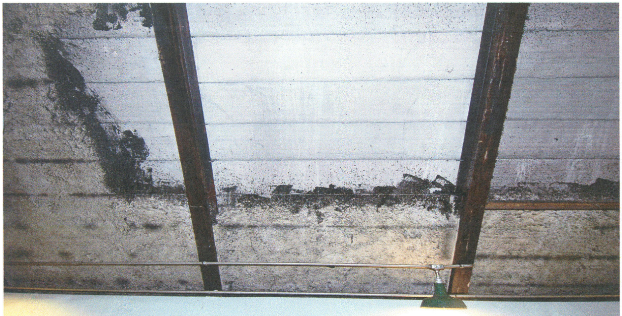
Asbestos has been scraped away from this area in the attic of Building 3.
