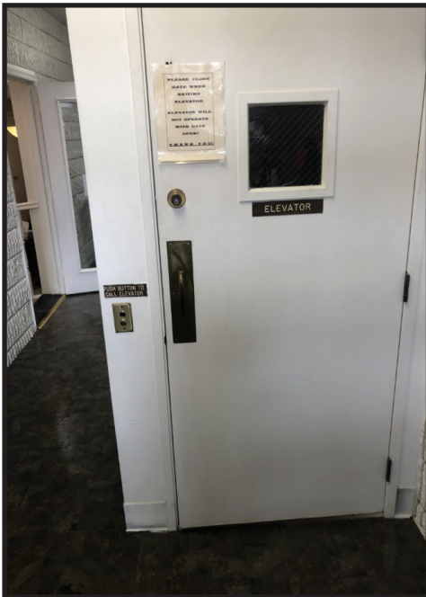
Picture 6 Elevator Exterior
