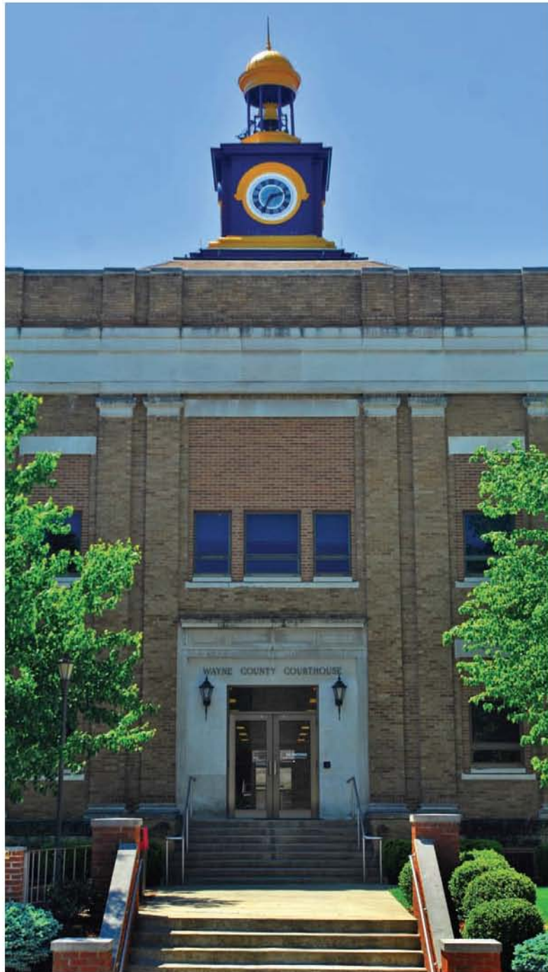
The Wayne County Courthouse in the town of Wayne opened in 1924 and was remodeled extensively in 1976. The structure is the fourth to be built for use as a courthouse. Its immediate predecessor burned in 1921, but records were preserved in a fireproof vault.
