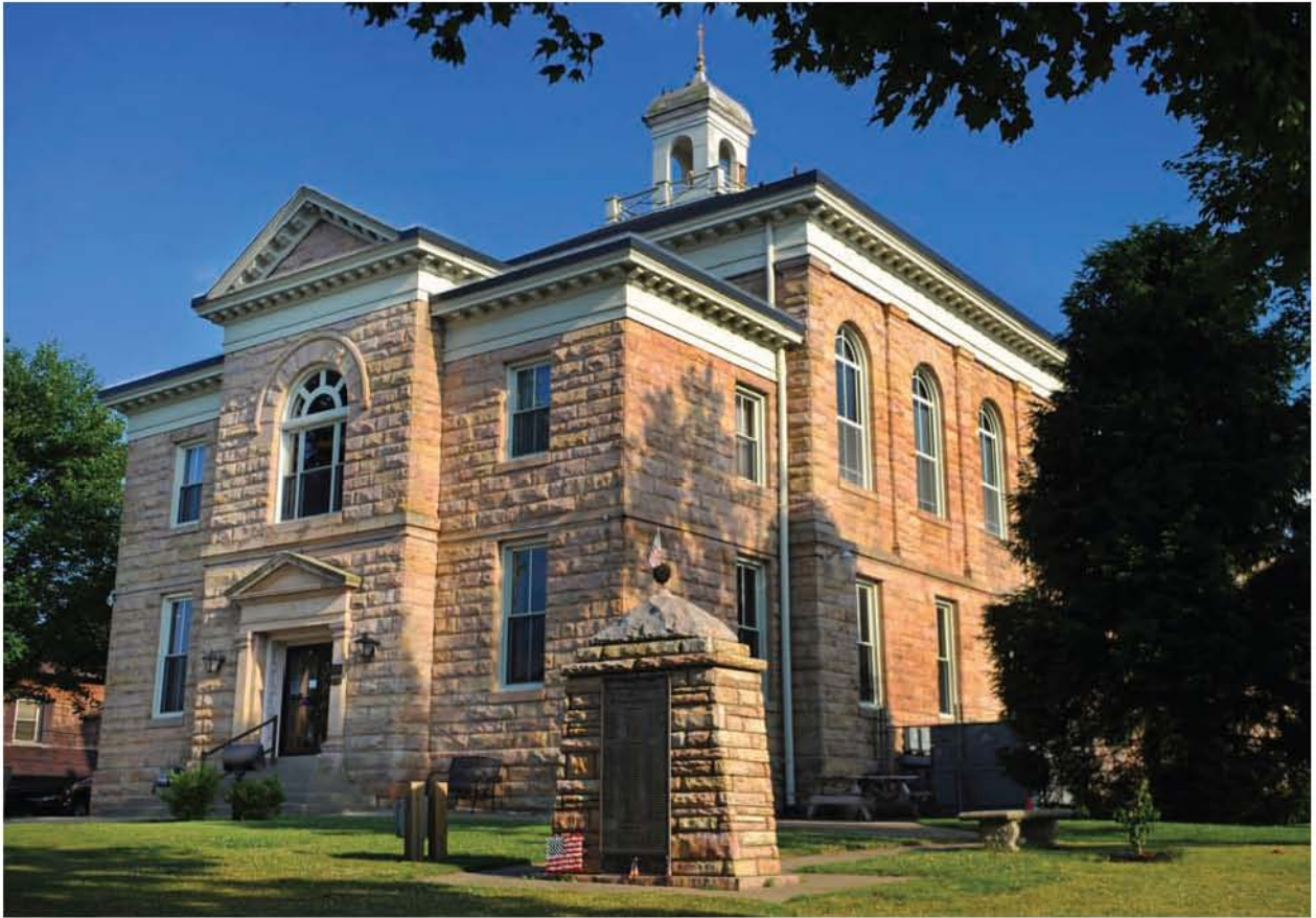
The Nicholas County Courthouse in Summersville was completed in 1898. The stone structure, the county's second courthouse, has a large bell in its cupola. The courtroom was completely renovated in 1998.
