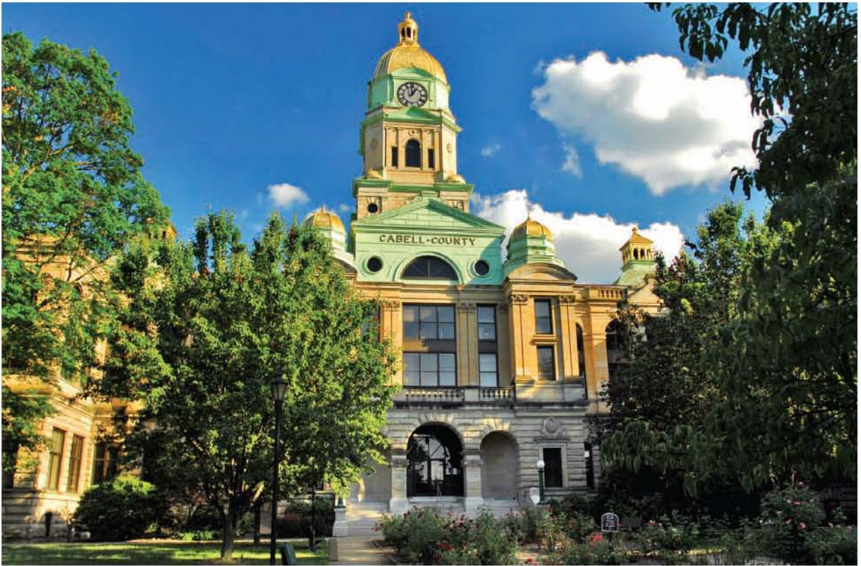
Construction on the Cabell County Courthouse in Huntington, built of Berea sandstone and topped with copper, was completed in 1901. Wings were added in 1924 and 1946.
