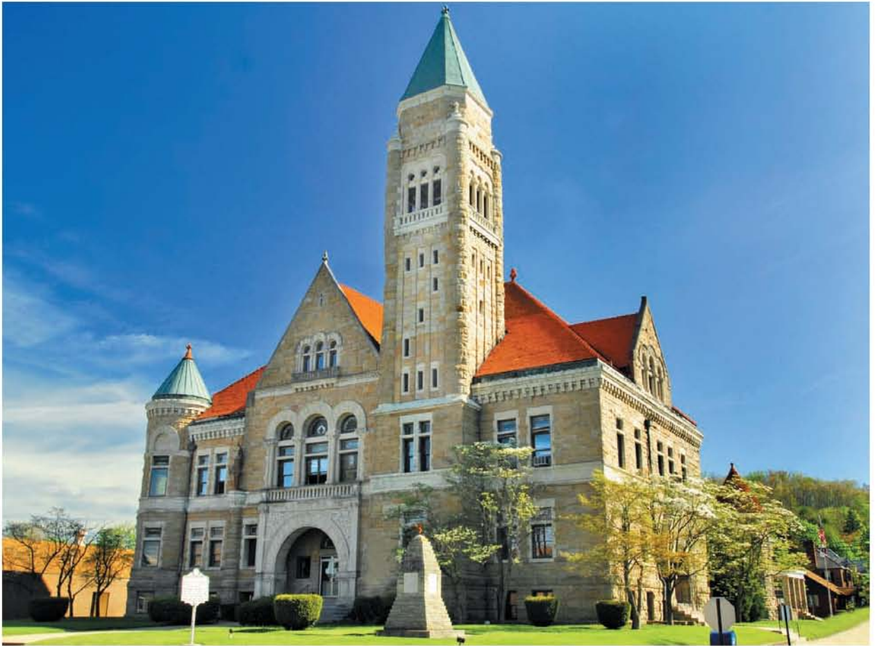
Randolph County's courthouse in Elkins was built between 1902 and 1906. It is made of hand-cut stone and decorated by stained glass. The building is the second in Elkins to serve as a courthouse. Three others in Beverly were previously used for court sessions.
