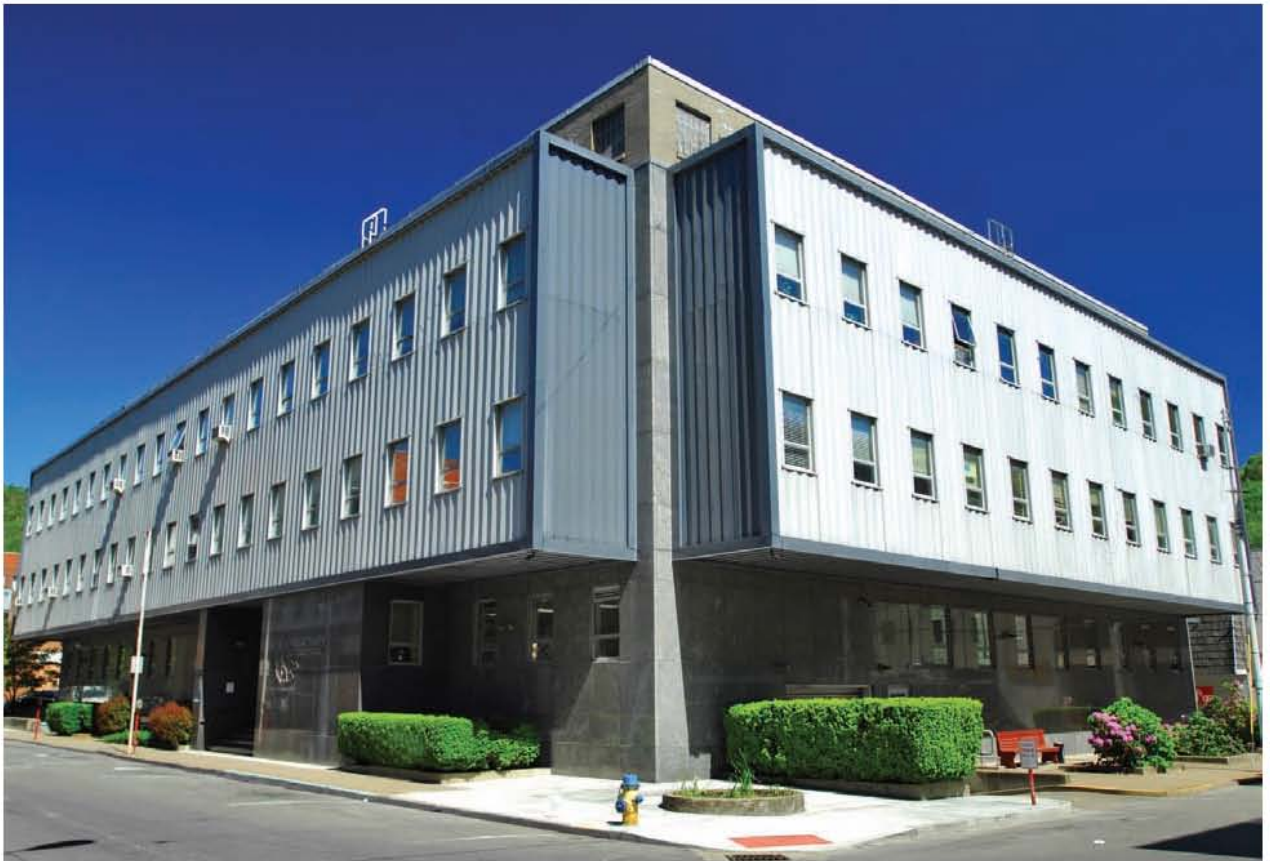
The Logan County Courthouse in the town of Logan was built in 1965, the fourth since the Civil War. An earlier structure was burned by Union troops, along with all records.
