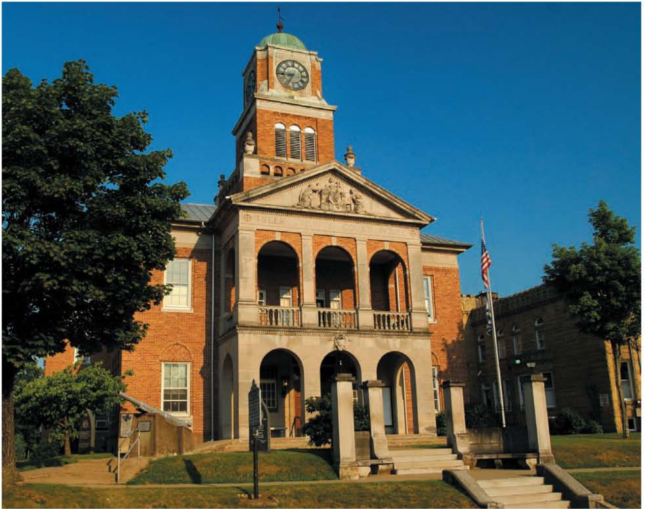
Tyler County's courthouse in Middlebourne was built in 1852 as the county's first permanent courthouse. It was expanded in 1922, when the original section and the new wing were both faced with identical brick.
