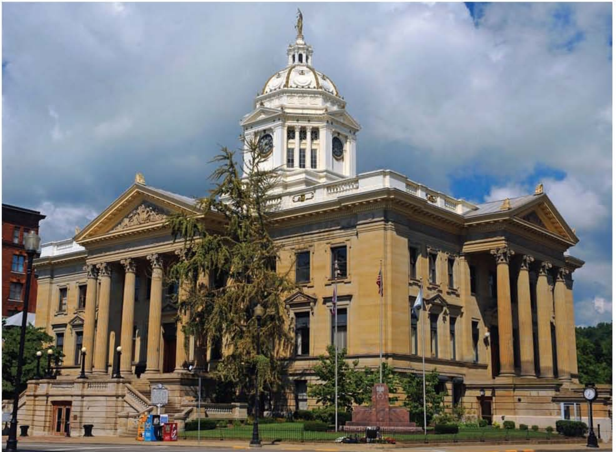
Marion County's courthouse was built in Fairmont between 1897 and 1900 of Cleveland sandstone. The county's second courthouse, it features a stained-glass dome in the third-floor courtroom.
