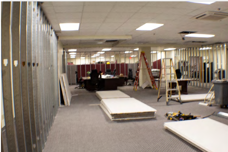
Construction begins on The Justice Center, our in-house learning studio to be completed in FY 2019.
