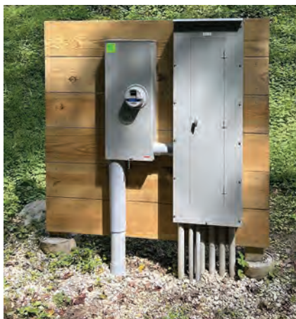
Kanawha State Forest Campground Electrical Upgrades
