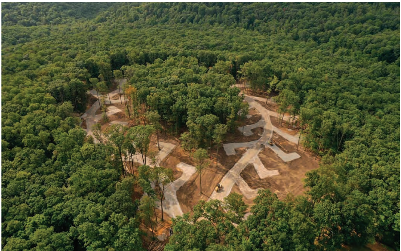
Coopers Rock State Forest Campground Addition in Construction
