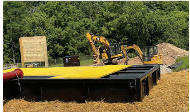
Beech Fork EQ Tank Replacement
