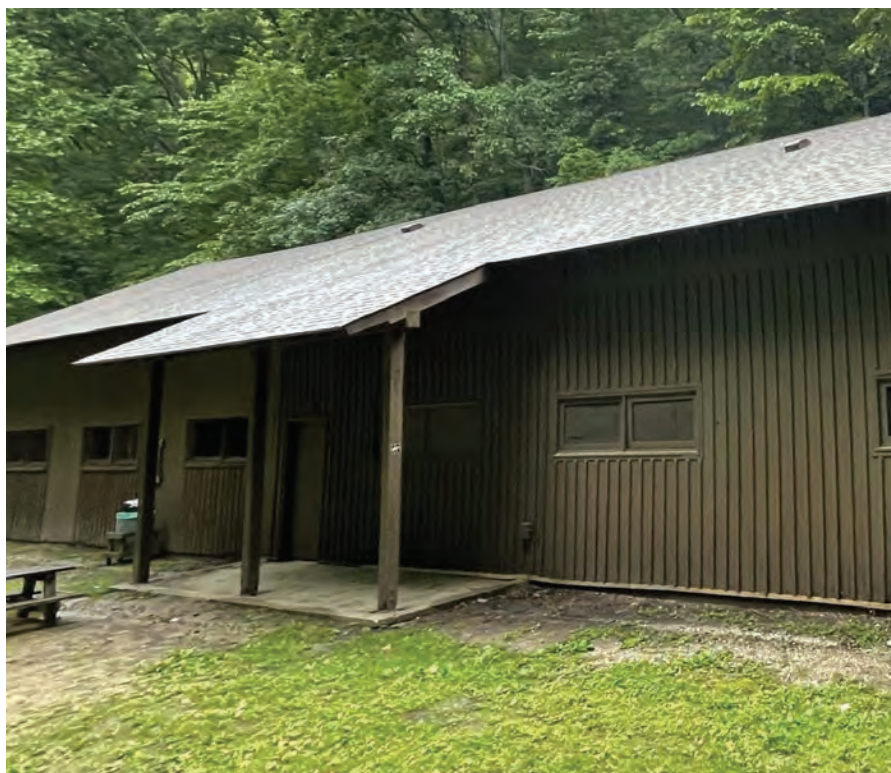
Kanawha State Forest Stable Roof
