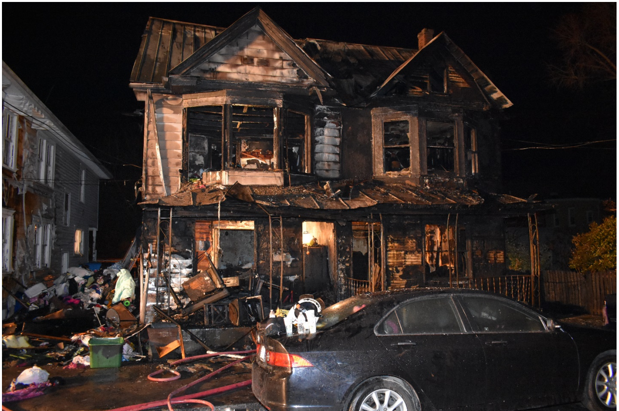
Berkeley County/Photo by ASFM Harms
