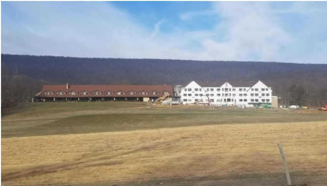
Cacapon State Park Lodge Addition
