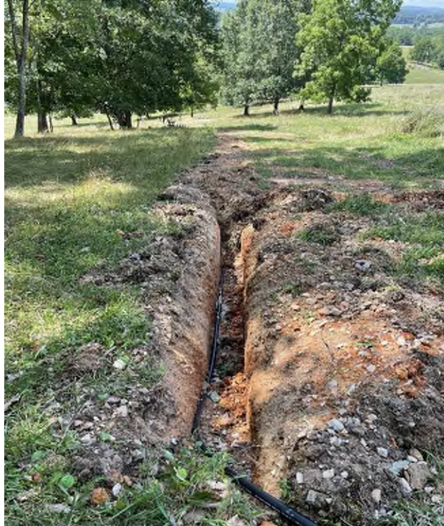
Pipeline for Watering System
