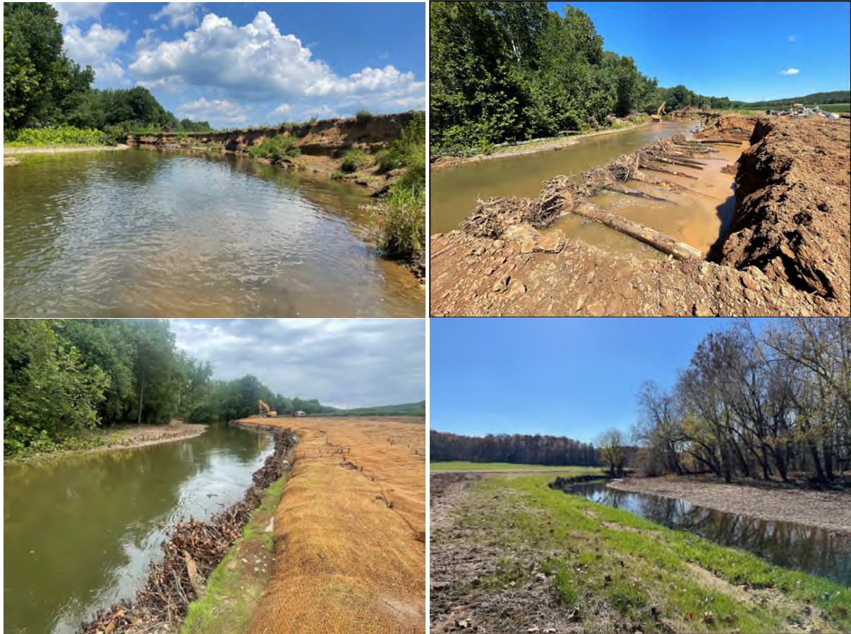
Back Creek stream restoration and bank stabilization September 2022
