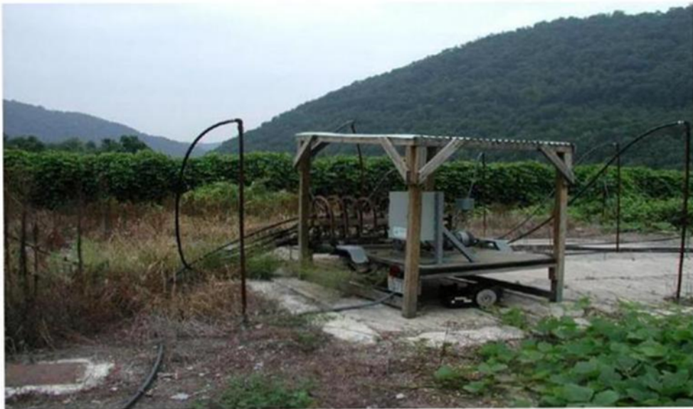
Employing air sparging at a groundwater cleanup site
