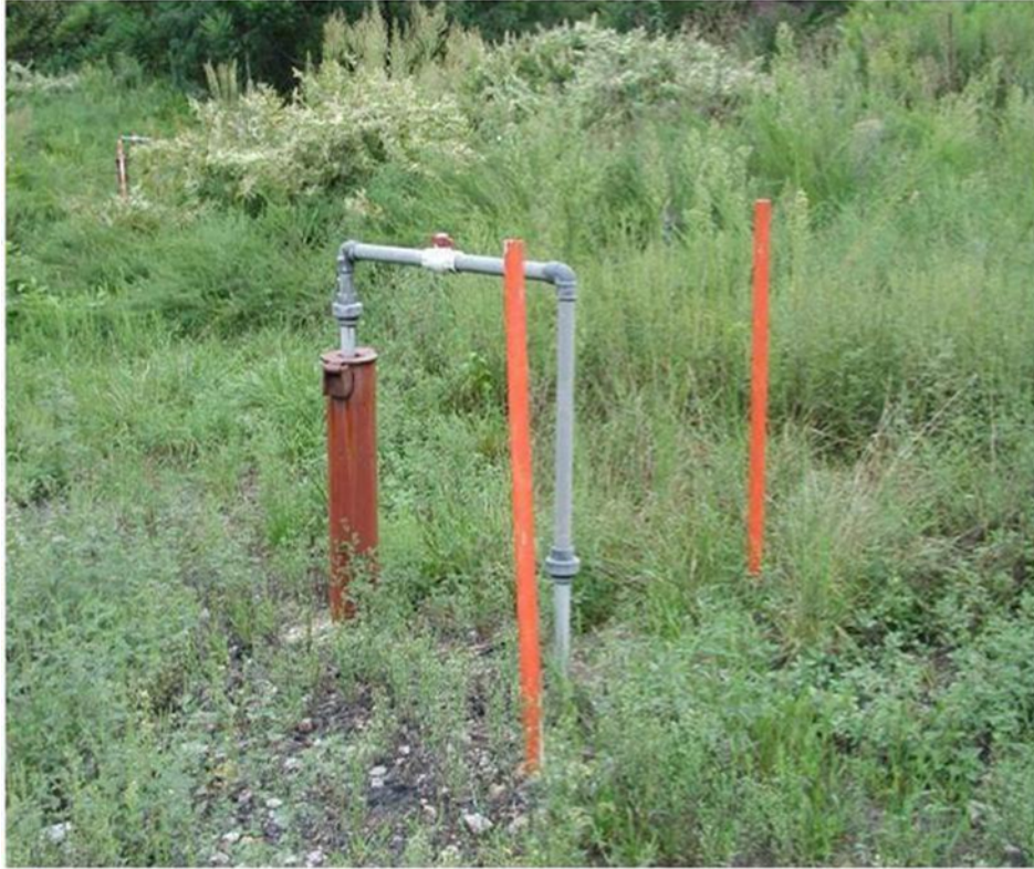
Employing bio-venting at groundwater cleanup site
