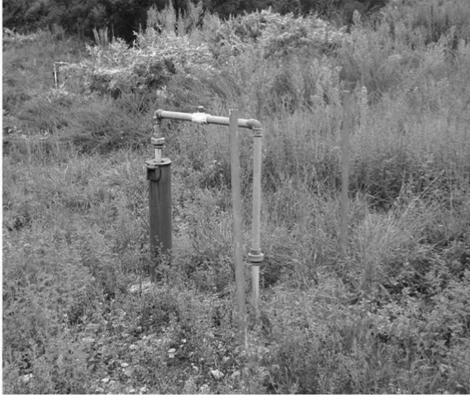
Employing bio-venting at groundwater cleanup site
