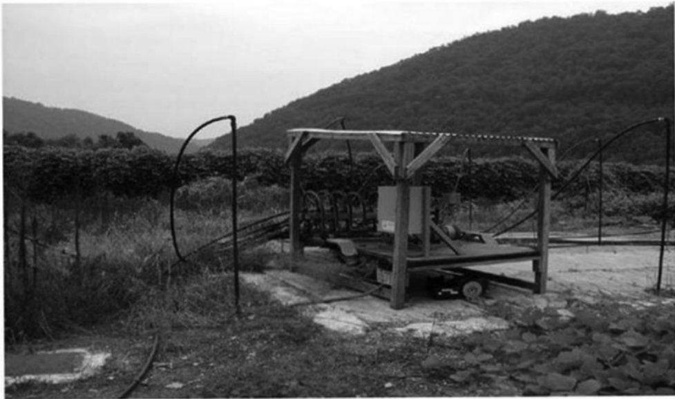
Employing air sparging at a groundwater cleanup site
