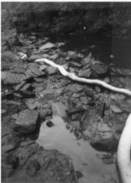
Hydrocarbon sheen on a stream with absorbent pads being used to keep the contamination from entering the stream.
