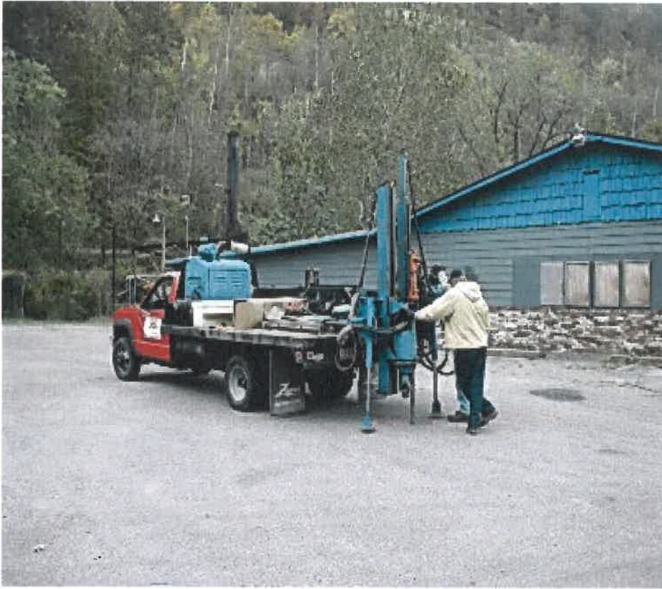
Above, a Geoprobe unit injects oxygen release compounds at a bio-remediation site. Below, a high vacuum pump truck extracts hydrocarbons.
