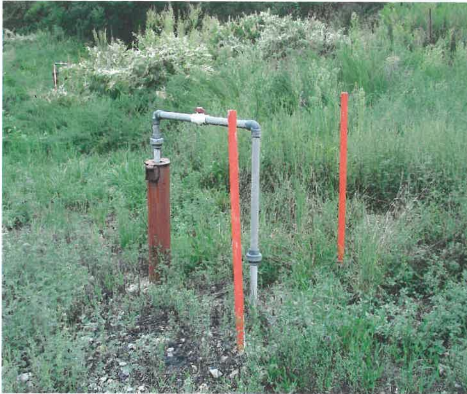
Employing bio-venting at groundwater cleanup site
