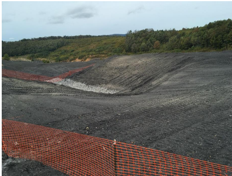
Figure 4: Completed test plot, 9/5/2017
