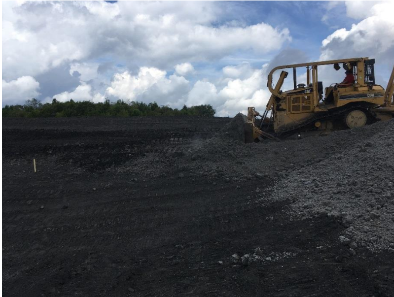
Figure 5: D-6 Dozer spreading residual material
