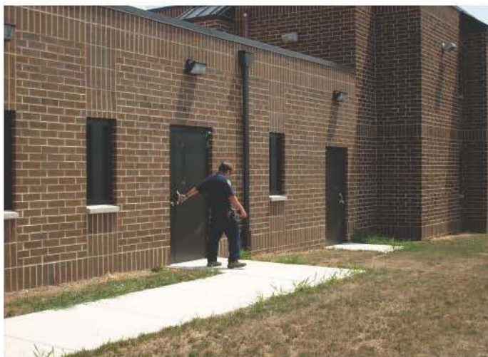
MCC's New Addition
