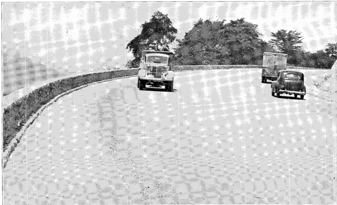
The Glendale Narrows, Formerly Regarded as the "Most Dangerous Piece of Road" in the State. This 1.6 Mile Section of Routes U. S. 250 and W. Va. 2, is Now a 44-foot Wide, Four-lane Highway
