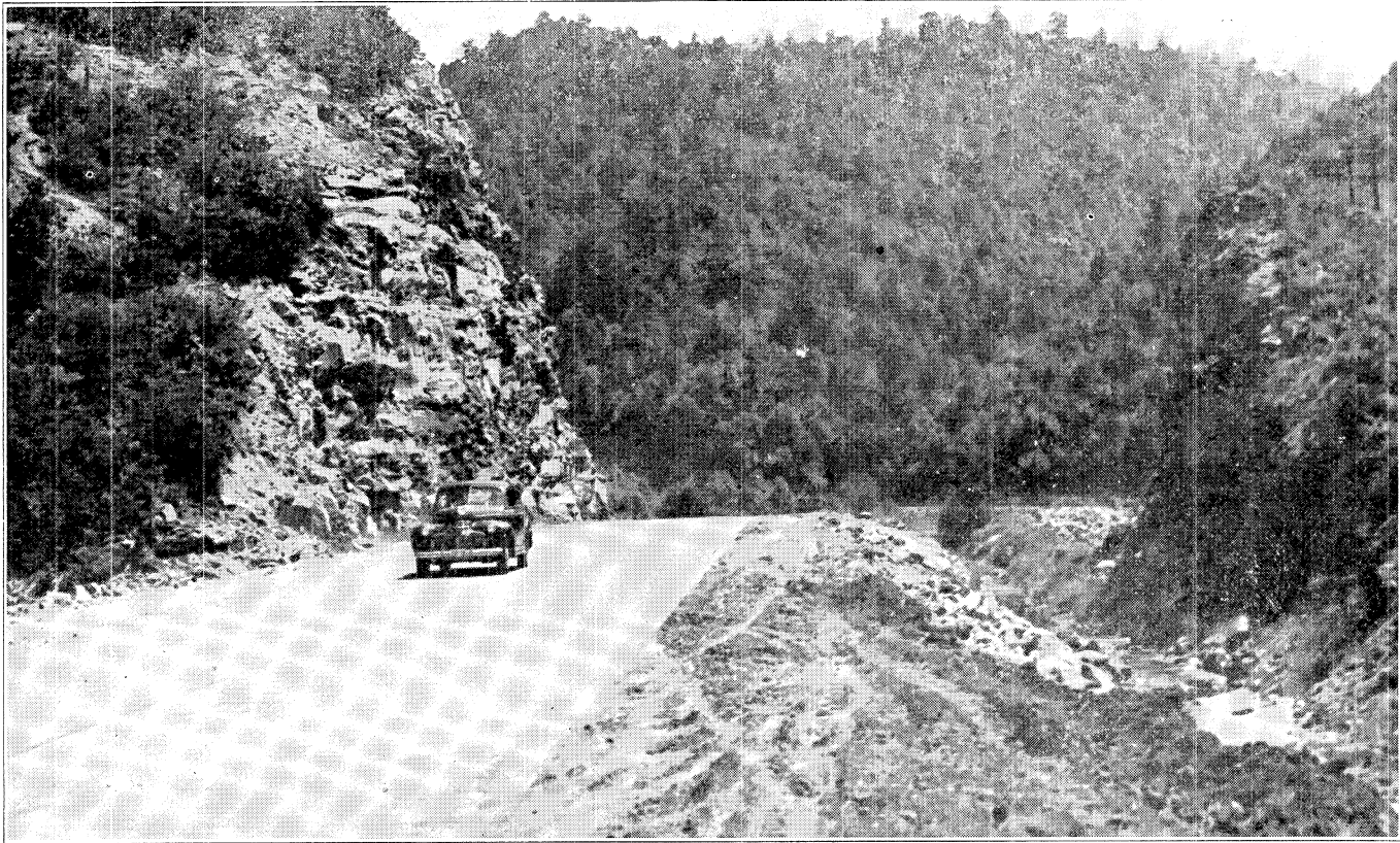
Cut Through a Mountainside on U. S. 52 in McDowell County.
