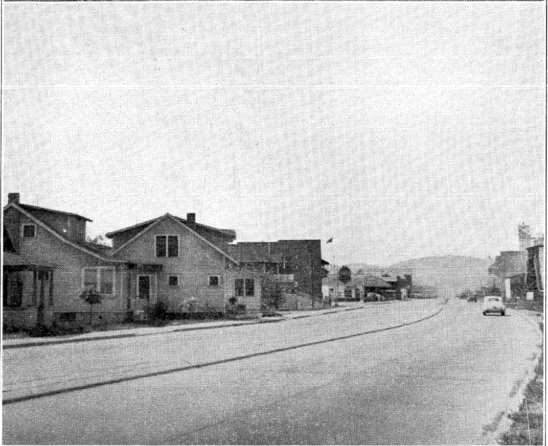
Access Road Development on U. S. Route 60 at South Charleston. Top picture taken from new $458,000 grade separation structure over railroad spur, looking east. Bottom, same road looking west. Four-lane divided highway designed to relieve congestion.
