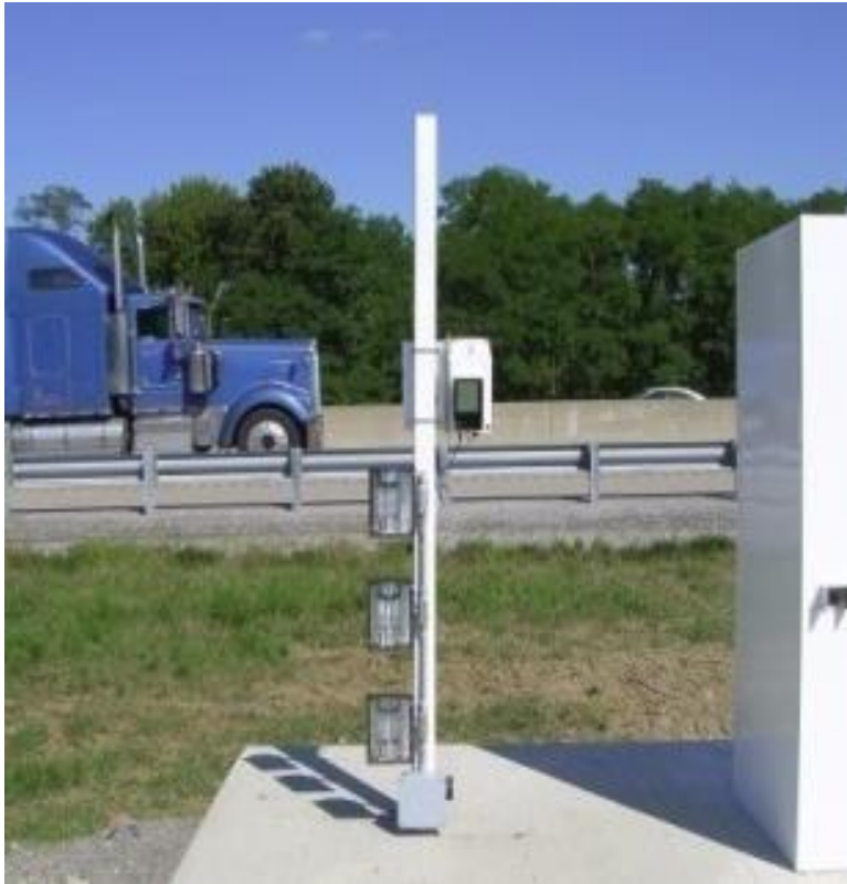
Virtual Roadside Inspection Station
