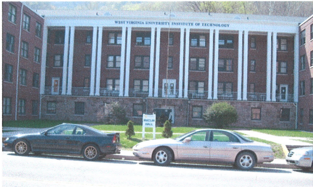
Figure 3: Entrance to Maclin Hall from Fayette Pike
