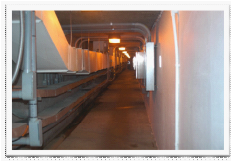
Underground Tunnel Beneath Toll Booth at Toll Plaza C
