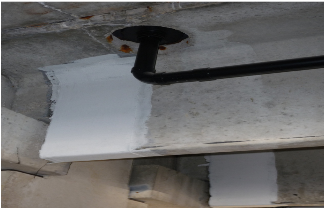
Figure 5 - A new roof drain has been installed to prevent water ponding.
