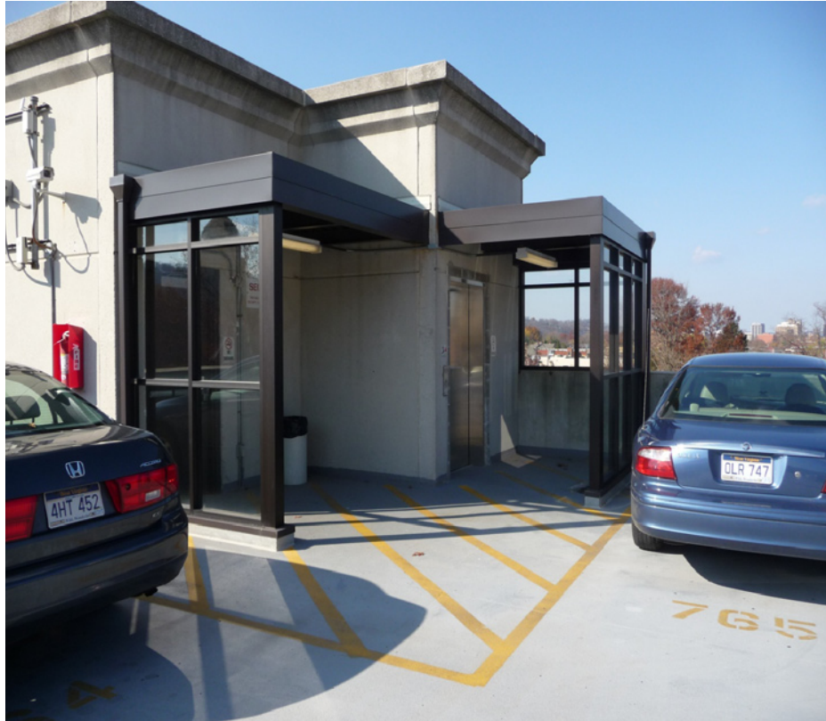
Figure 9 - New roof deck elevator enclosure to reduce water damage to elevators.
