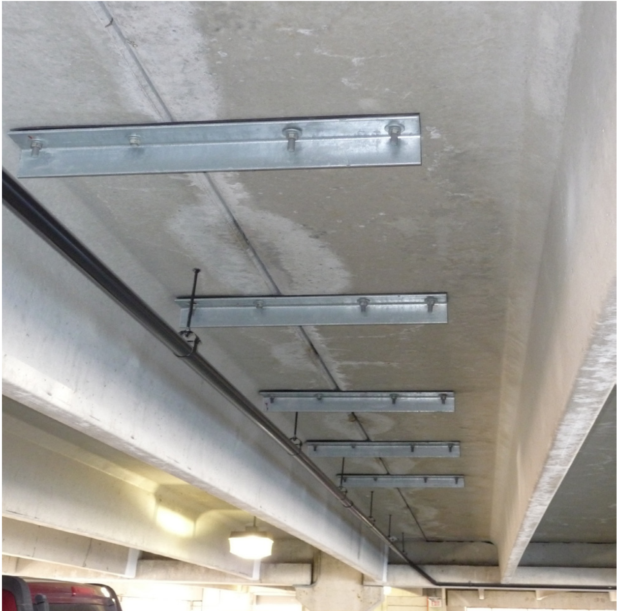
Figure 8 - New ramp deflection supports to minimize deflection between precast panels.
