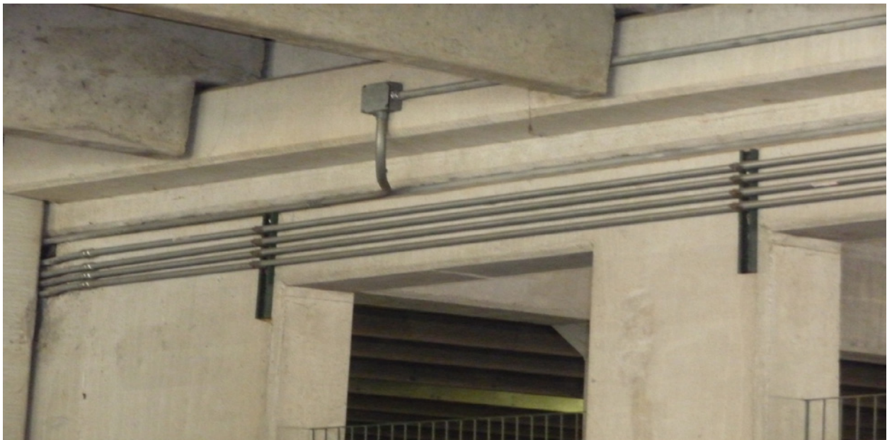
Figure 7 - Replaced electrical conduit and supports.
