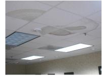
Figure 6 - Areas of leaks on top floor of Building 86
