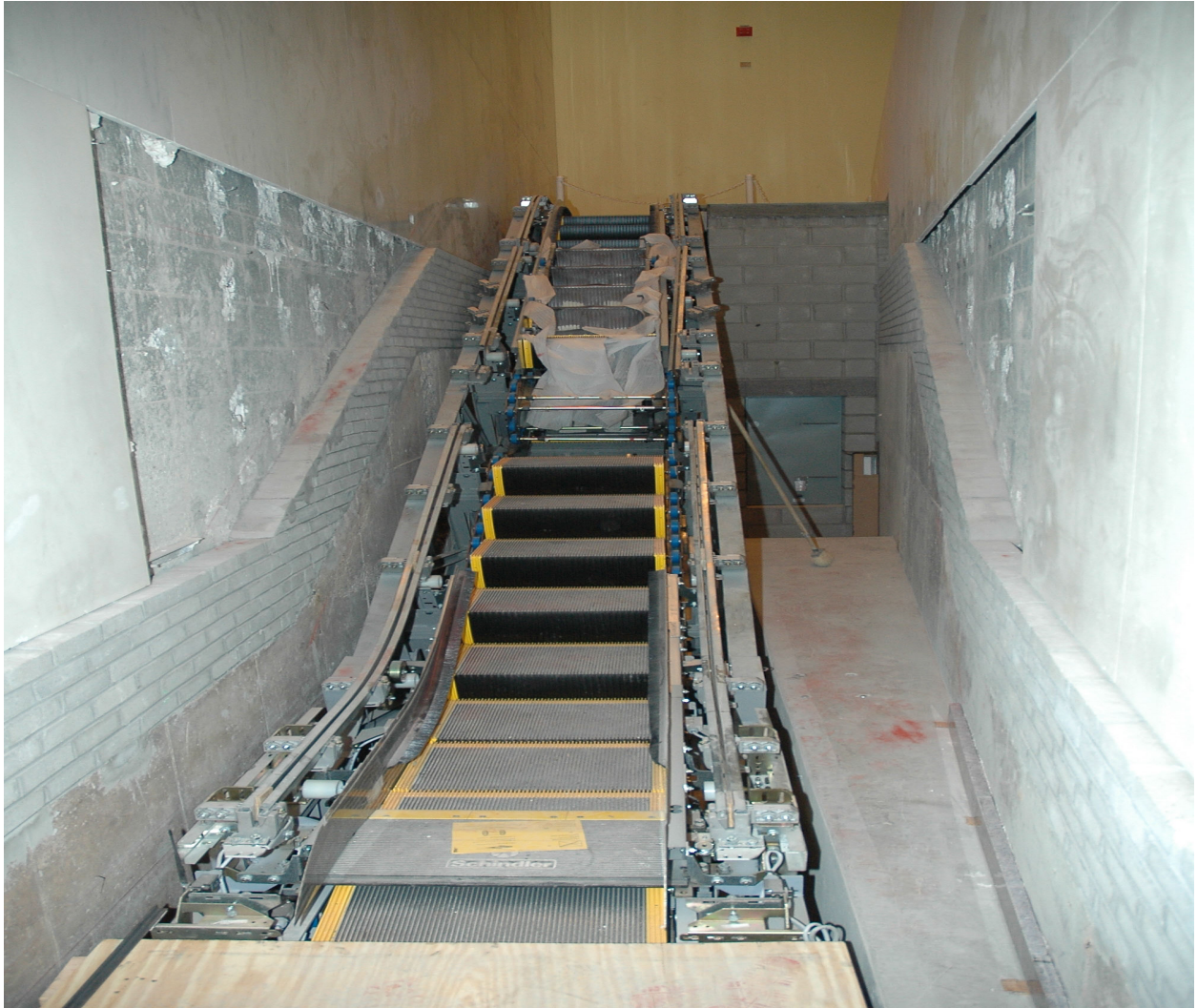
South escalator under installation.
