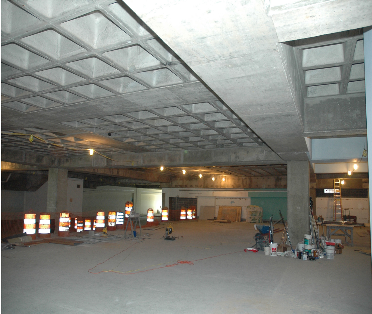
Main museum looking toward south end of building.
