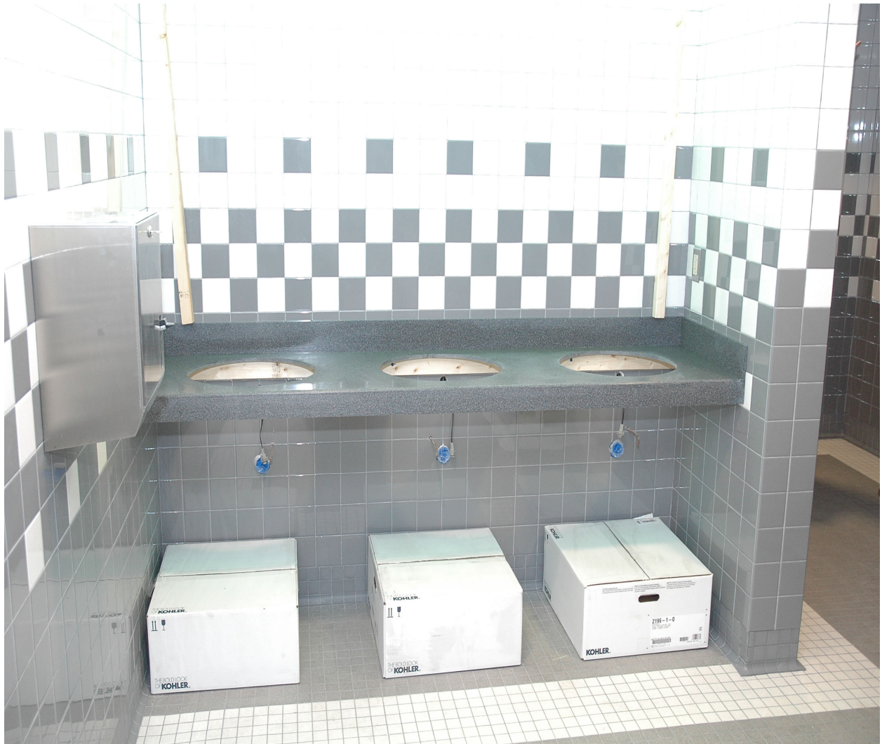
New restroom which has ADA compliant facilities.
